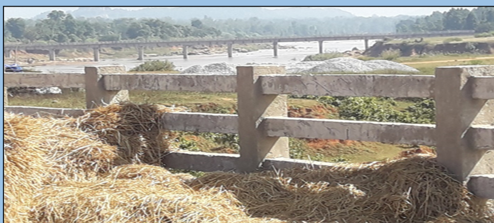
Picture 2.2: Incomplete MMGSY bridge and complete PMGSY bridge at a distance of about 500 m at Khursurta and Bardih in Gumla district (Joint physical verification done on 19 November 2019)
