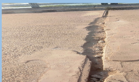
Picture 2.18: Absence of expansion joints in bridge across Swarnrekha river between Khokro-Karkidih road in Ichagarh block of Saraikela district
