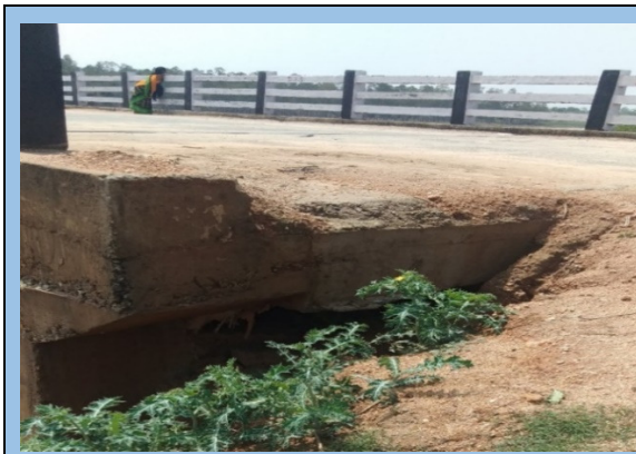
Picture 2.16: Washed away approach in the flank near approach slab in bridge across Amanat river between Saraiya-Jhalkhandi, block Panki of Palamu district
