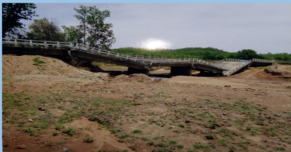
Picture 2.8: Photograph of collapsed bridge over Charki river between Natwal-Dina Road .)
