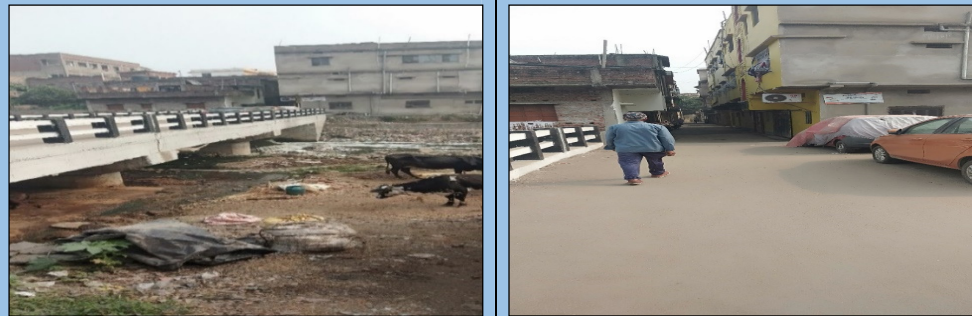
Picture 2.4: MMGSY bridge in urban area of Dhanbad city and existence of buildings in the alignment of bridge (Joint physical verification done on 27 November 2019)
