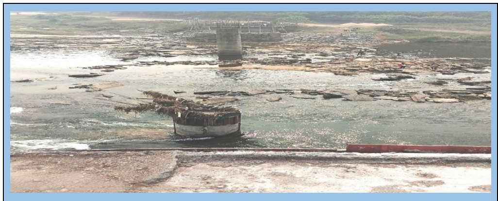
Picture 2.15: Partly constructed substructure P9, P11, old A2 (to be dismantled) and under construction A2 in bridge over Damodar river between Gansadih-Suyiadih road in Dhanbad
