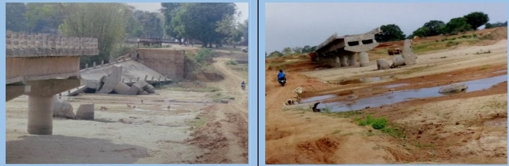
Picture 2.9: Photograph of collapsed bridge over South Koel river between Balkhatanga-Lorengo road in Sisai block
