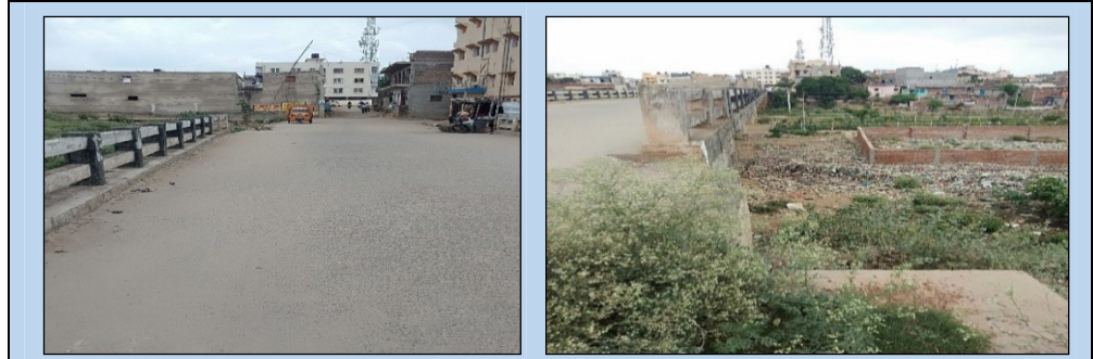
Picture 2.5: MMGSY bridge in urban area of Ranchi city and unauthorised construction under the bridge (Joint physical verification done on 20 March 2020)
