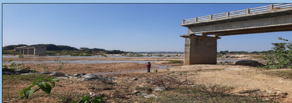
Picture 2.3 : Incomplete MMGSY bridge at Khursurta and Bardih in Gumla district from a different angle
